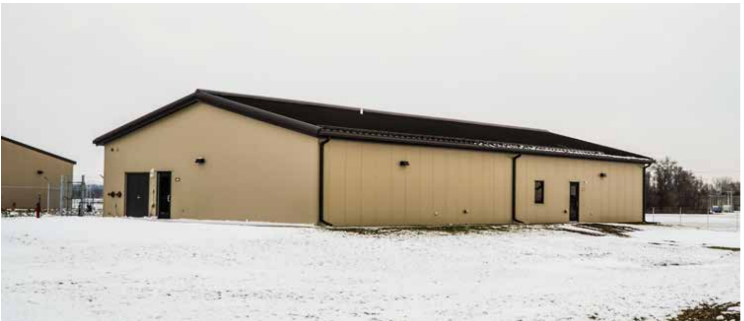
A new building for Detachment 1, 139th Medical Group, is near completion at Rosecrans. Det. 1 is responsible for the medical support of the Missouri National Guard's Homeland Response Force. The construction is part of a long term plan of moving the base north of its primary location. (U.S. Air National Guard photo by Master Sgt. Michael Crane)
